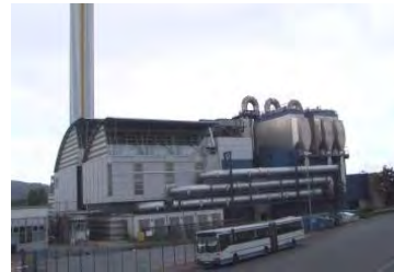
Waste Incineration Plants
